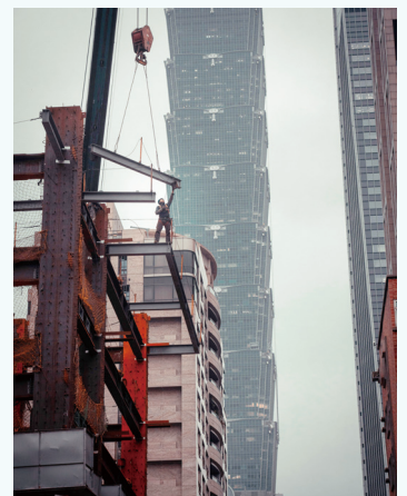
COVER PHOTO BY JIMMY LIAO FROM PEXELS. CONSTRUCTION WORKER STANDING ON STEEL BEAMS IN FRONT OF TAIPEI 101.
